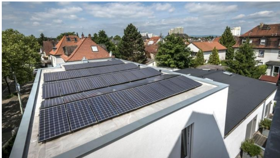
Example of solar panels installed on a flat roof
